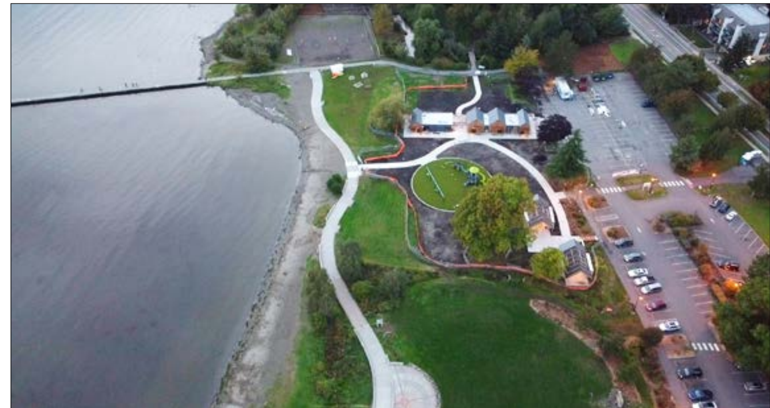
Construction forced the City to close part of Juanita Beach Park to the public. However, it kept open many of the park's other features, including its walkways, its beach, volleyball courts and its grassy lawns.
