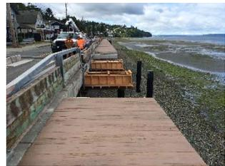
At typical high tide, the Redondo Boardwalk experiences overtopping saltwater waves making the use of typical cast in place concrete very difficult. Utilizing precast decking provided the durability of concrete without risk of failure that cast-in-place concrete would suffer. Using this method was widely accepted by stakeholders for whom durability and reliability was important.
