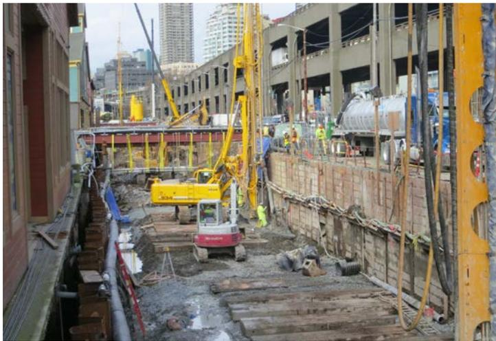
*Installing improved soil mass (ISM) foundation by jet grouting*
