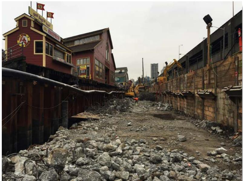
*Before - - Demolition of existing seawall, shoring wall on right, containment wall and Pier on left.*
