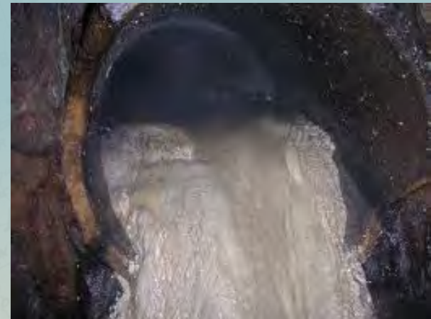
Grease on walls of a sewer pipe
