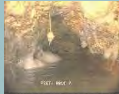
Grease on walls of a sewer pipe
